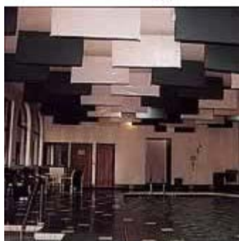
Example of a room ceiling with sabins absorption panel
